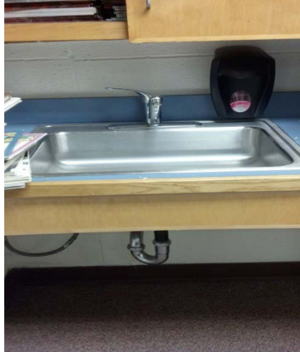
Existing ADA Sink
